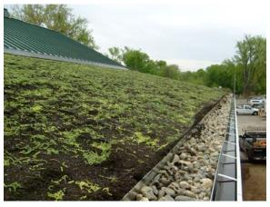
This green roof project involves a 13,000 square-foot area with a 25 percent slope. Design includes sturdier roof framing, a thick waterproof membrane to protect the roof, and four inches of bio-engineered growth media that is planted with eight varieties of Sedum to reduce stormwater runoff from the roof. In addition to capturing rainfall, the roof improves energy efficiency within the building, lowering heating and cooling costs.
